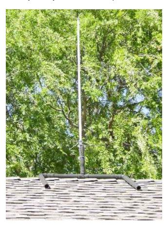
This mount won't be good for tall masts, unless it is guyed. But is an easy way to get the antenna up on the roof, if only temporarily.
