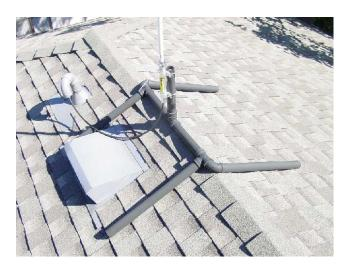
As can be seen in the photo, the mount is made up of four two foot sections ("legs"), three one foot sections (two along the ridge, one vertical), three tees and two 90 degree elbows.
